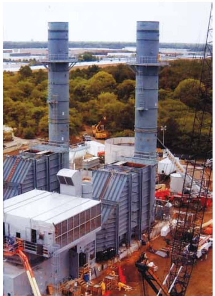
79.9 MW natural gas-fired simple cycle Edgewood facility in Brentwood, NY, one of two power projects built using DiFazio teams. The other is oil-fired and is in Shoreham. Both plants have recently been acquired by J-POWER USA and the John Hancock Life Insurance Company. Both are fully contracted to the Long Island Power Authority.
